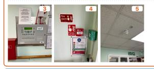
A hardwired, Grade A Fire Alarm system has been provided to the property with detection equipment provided within the communal areas and interlinked detectors within the flats.
